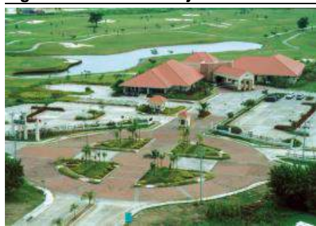
Fig 12 - Horizontal Project – Lakewood City
